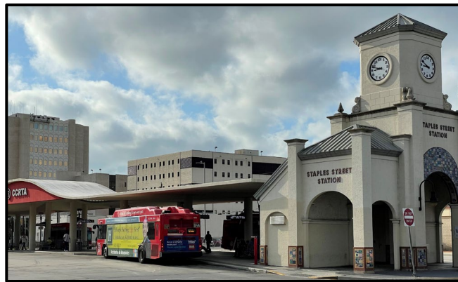
Figure 8 - Staples Street Station
