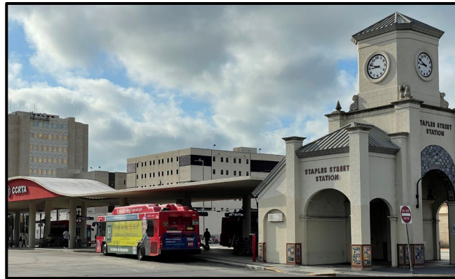
Figure 8 - Staples Street Station
